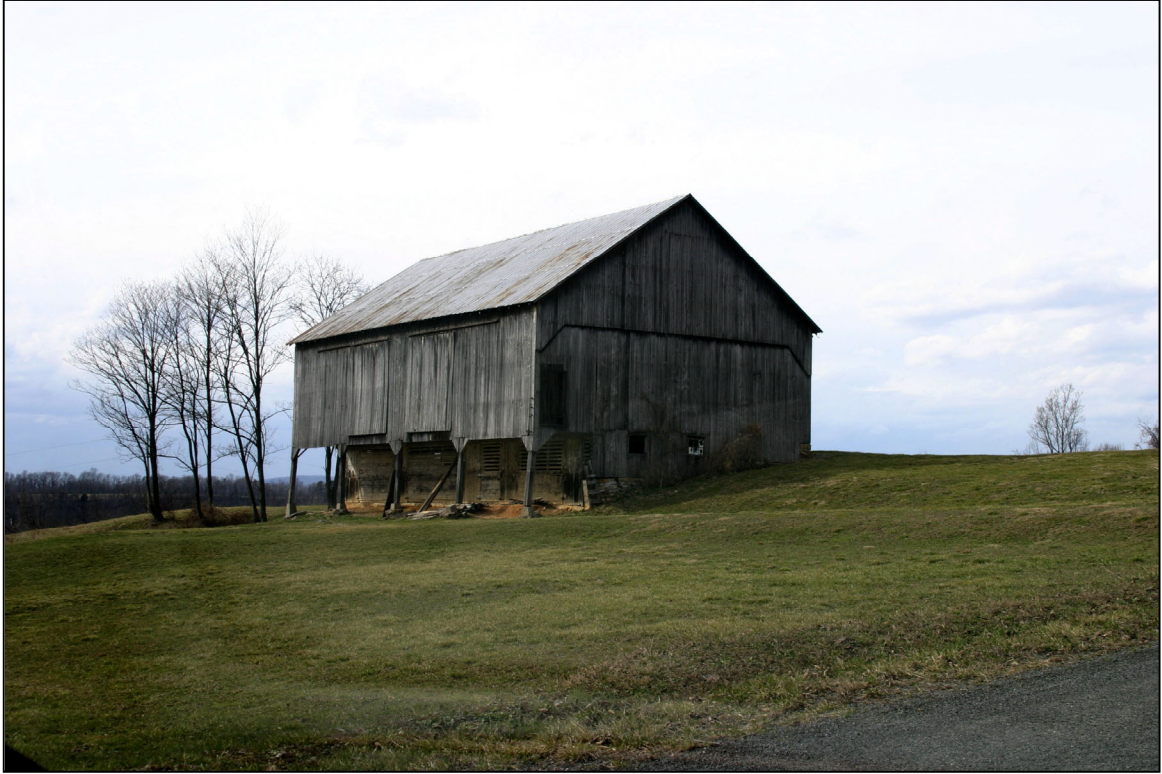
Figure 3.6. Pennsylvania Barn. This barn shows a typical overhanging forebay and banked entrance on the reverse side. Source: Author, 2003.
